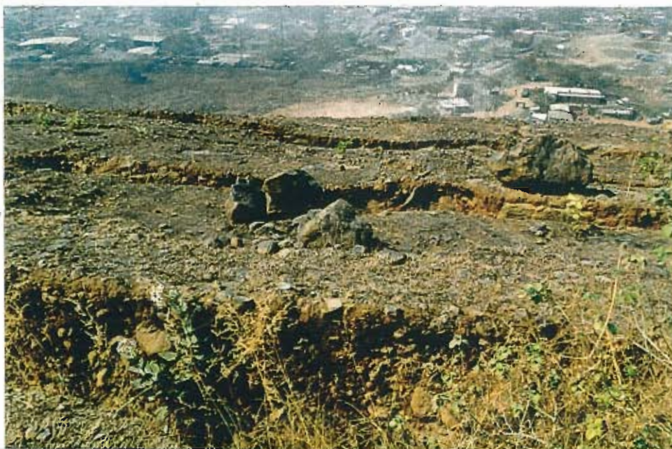
32. Cracks Observed Due to Quarry Operations Near Malad Forest Boundary
