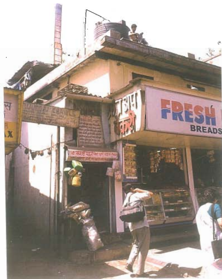
Plate No.6 Chimney Emerging out of Building
