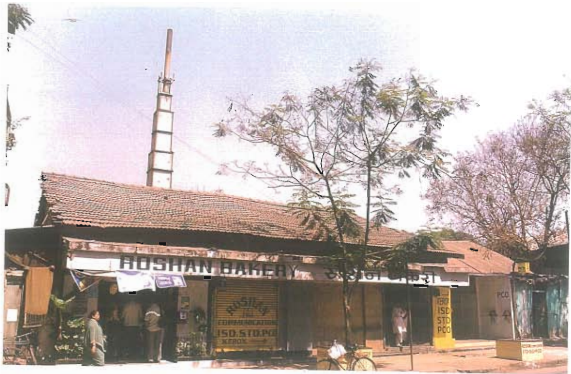
Plate No.5 Typical Chimney
