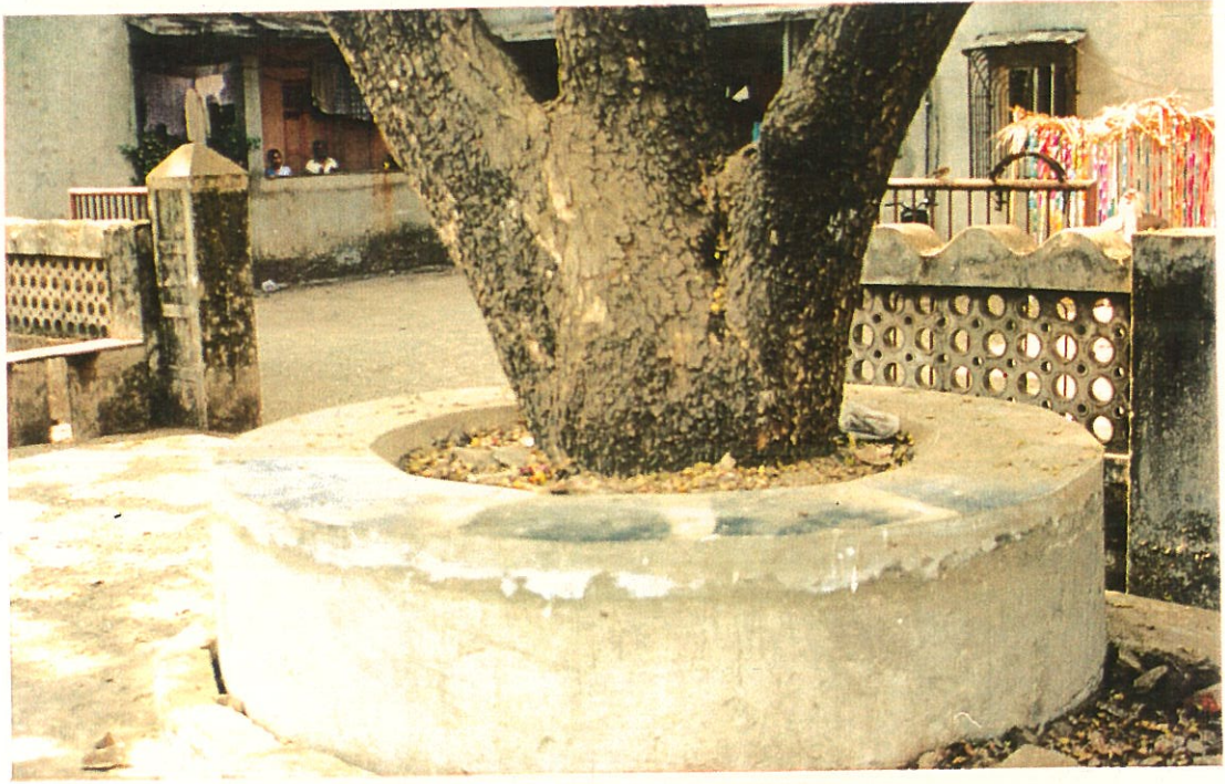
5.12 A proper tree base providing root aeration & irrigation, Subhash Nagar, Chembur
