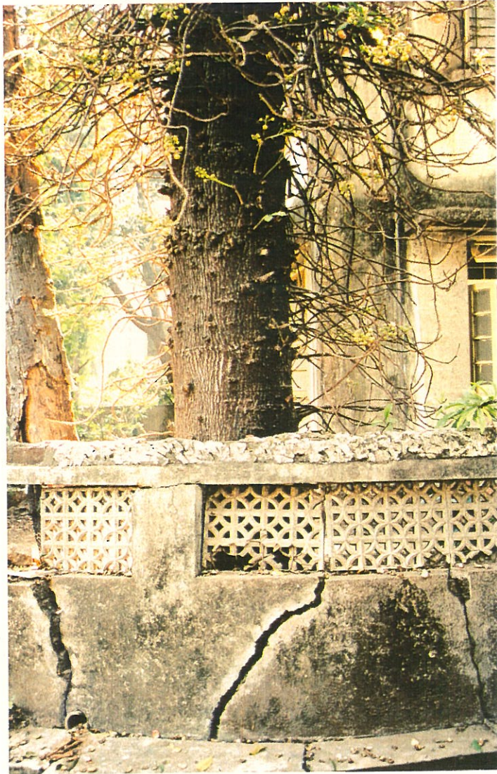
5.11 Kailashpati tree very close to compound wall is unsafe for the structure
