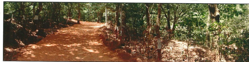
CULVERTS NEED TO BE PROVIDED ALONG ROAD IN THIS AREA TO CARRY WATER FROM THE CATCHMENT AREA INTO THE STREAM AND PREVENT SOIL ALONG ROAD BEING WASHED AWAY
