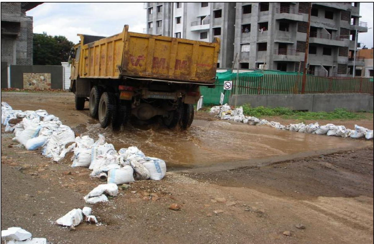
Picture No. 3-2: Water pit at entry and exit points for washing of truck tyres
