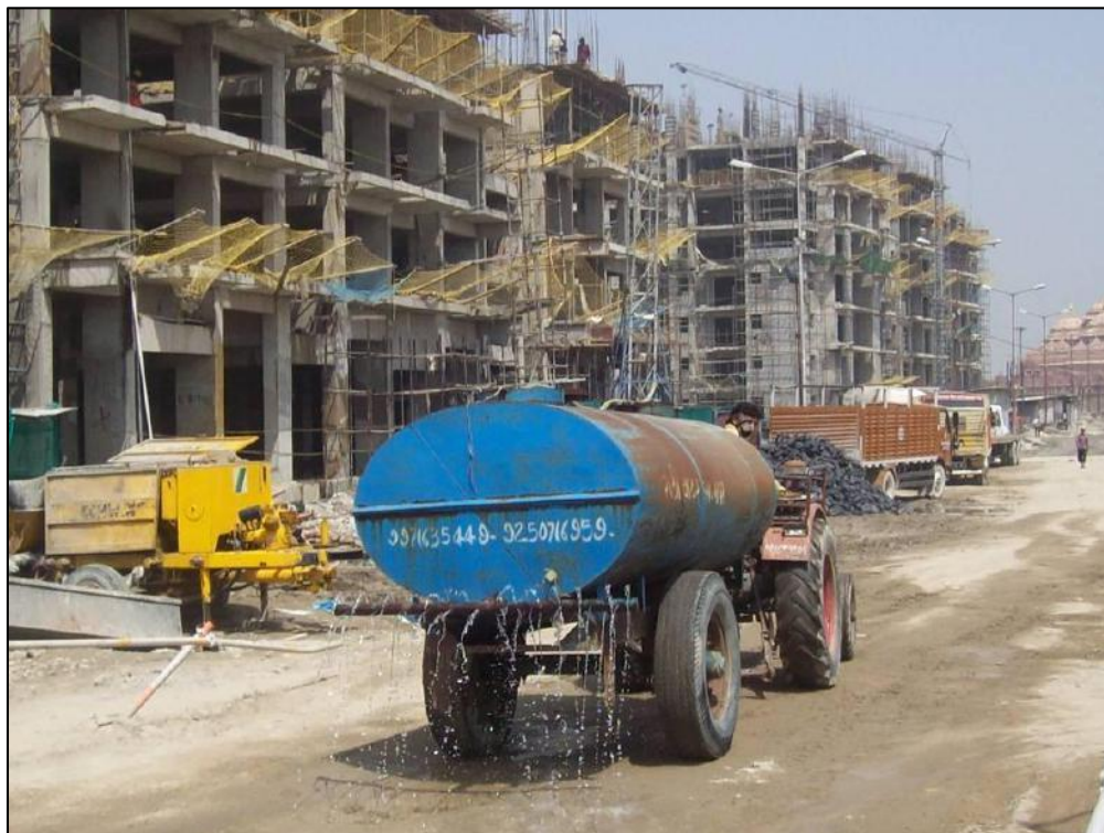
Picture No. 3-3: Sprinkling of water to reduce dispersion of dust at the construction site
