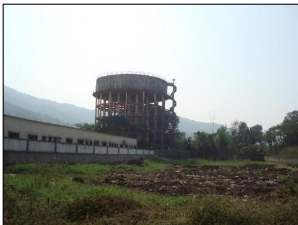
Picture No. 2-23: Overhead water filtration tank
