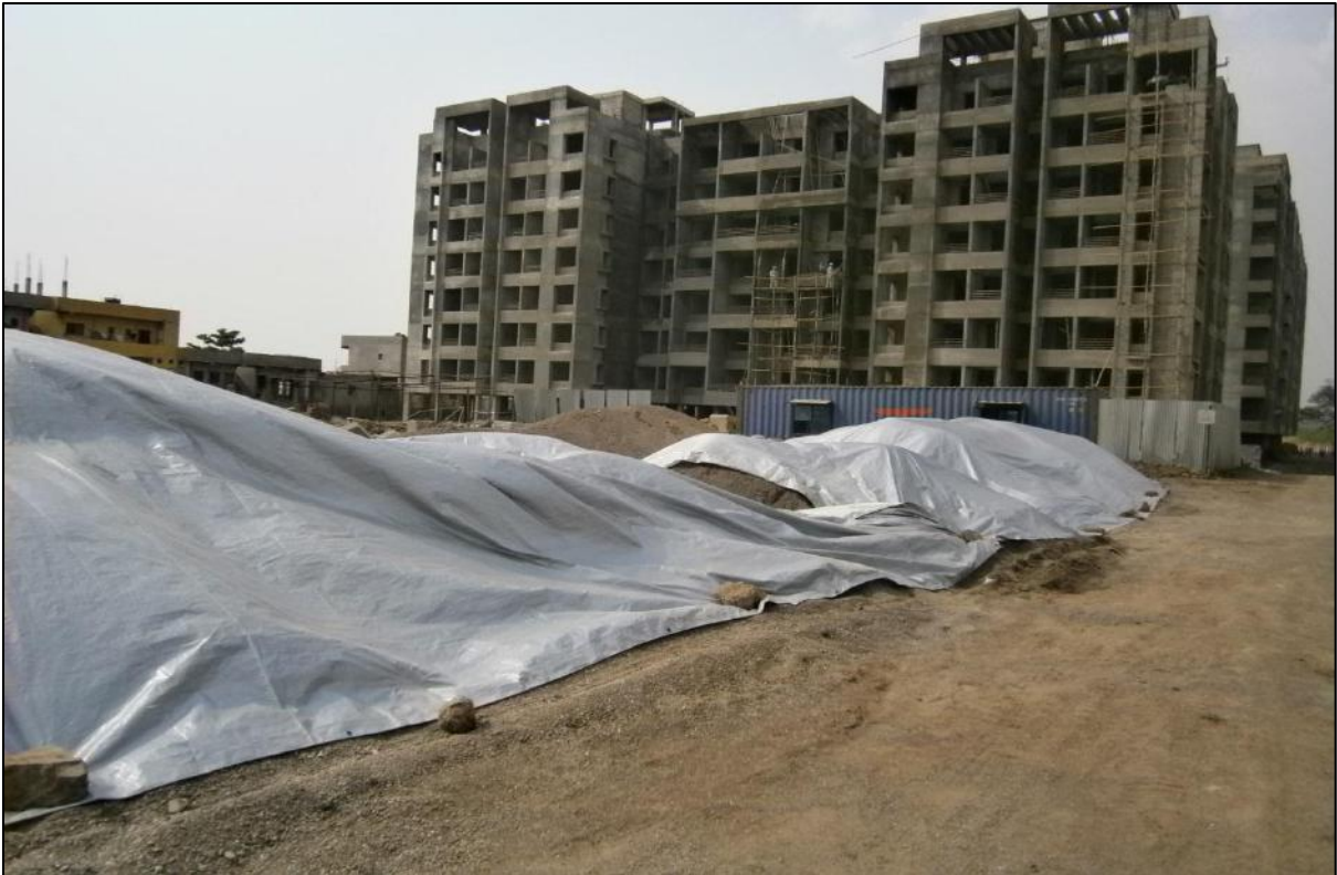
Picture No. 3-1: Covering of sand at a construction site
