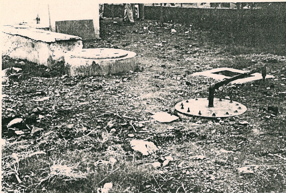
NBP Toilet Complex installed at Bhimad.
