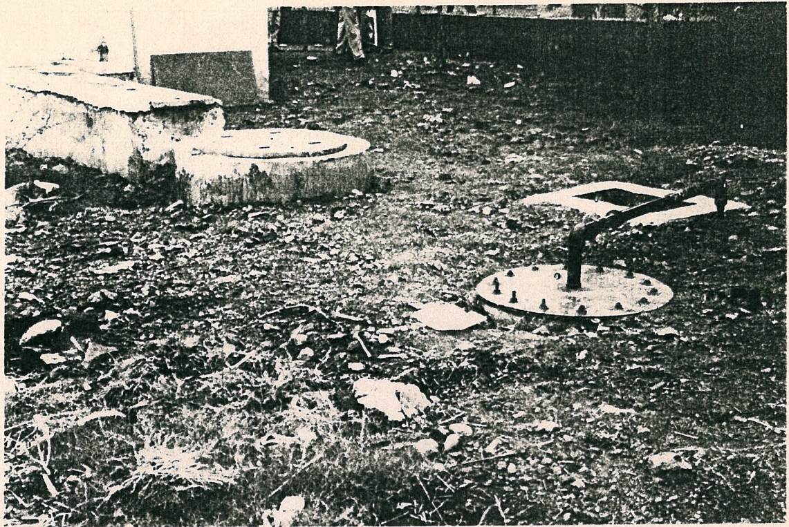
NBP's toilet Complex installed at Pshurani.
