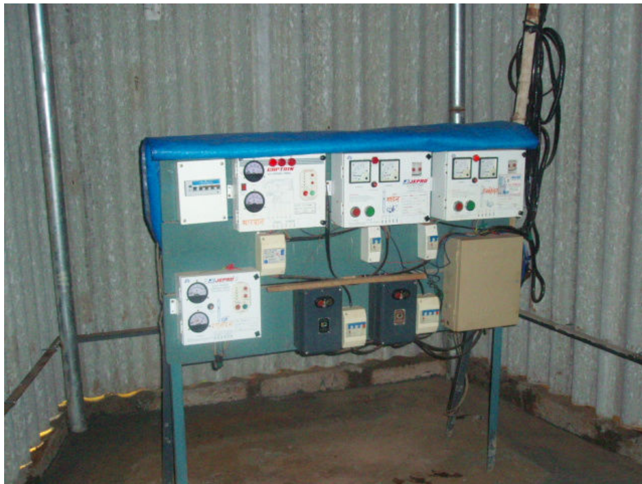
Treatment Plant Panel Board
