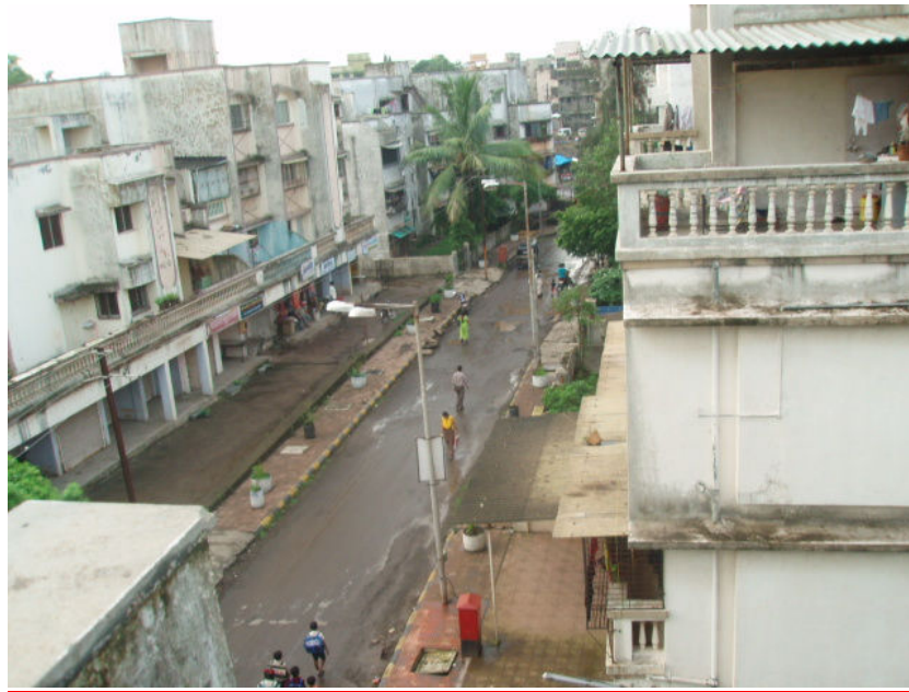
Actual Rain Water Harvesting Site "ShivDarshan Society", Kulgao Badlapur, Dist- Thane
