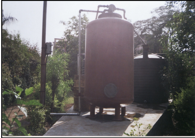
Filtration system for Rain Water
