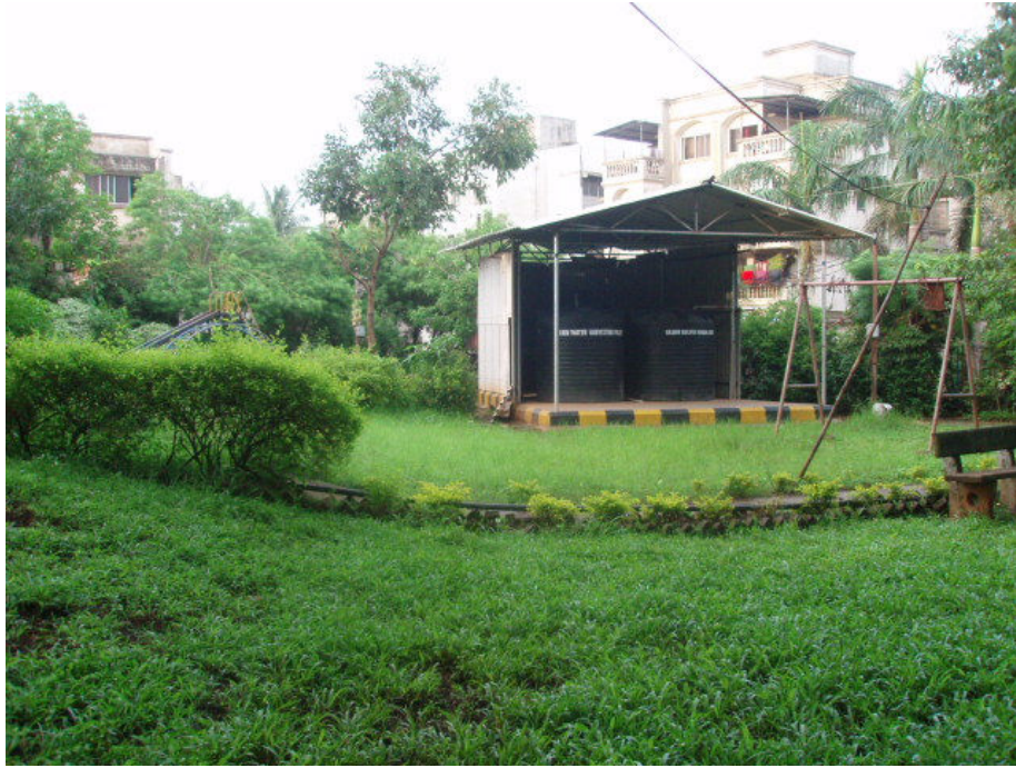
Rain Water Harvesting Treatment Plant
