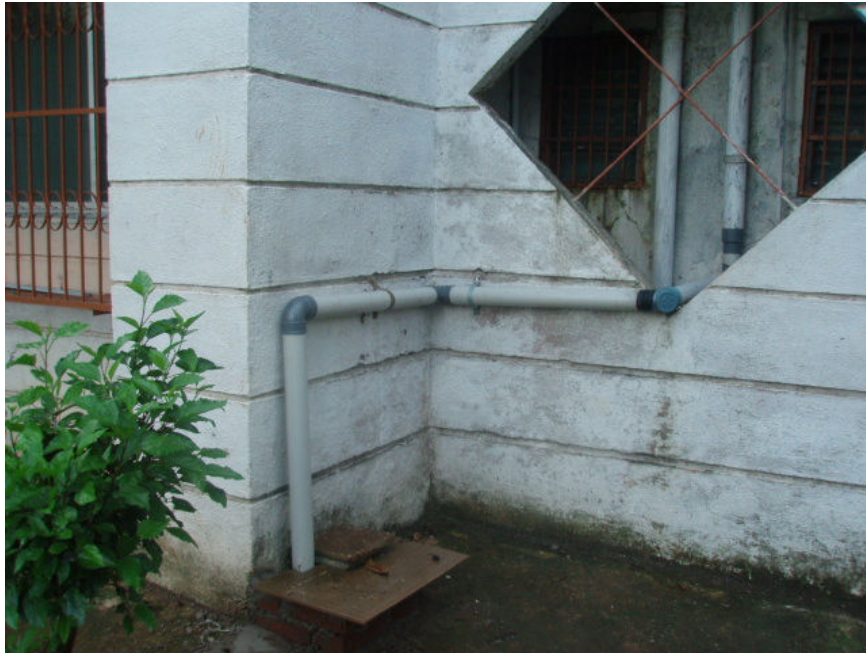
Diversion of Rain Water Down take pipe to Rain Water Harvesting Unit
