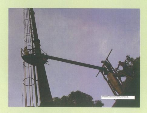
S.S. Dry Cyclone Separator was connected to the M.S. 30 Meters tall self supporting chimney by means of M.S. ducting as above.
