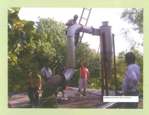
The refractory castable lined M.S. sections were provided on to the furnace. They came out on to the terrace as above. S.S. 304 Dry Cyclone Separator was erected in between the furnace outlet and chimney as above
