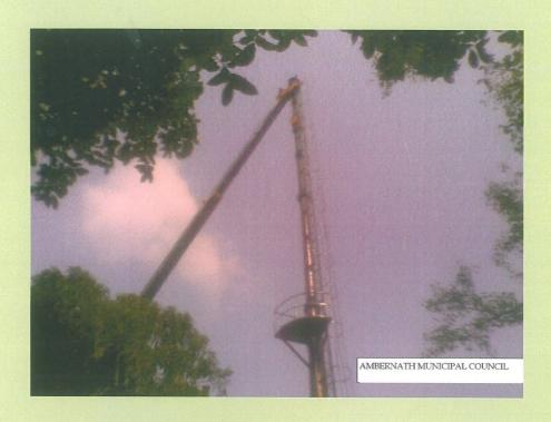
After 21 days curing of the R.C.C. block the M.S. 30 Meters tall self supporting chimney was placed in position by using telescopic Crain.
